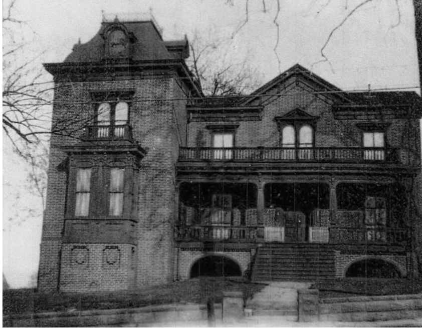
Haden Property, Park Street
