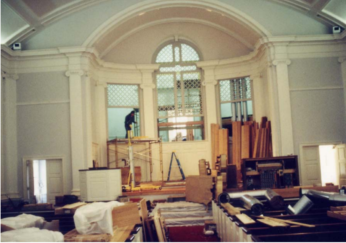
Installation of new organ, ca. January 1995
