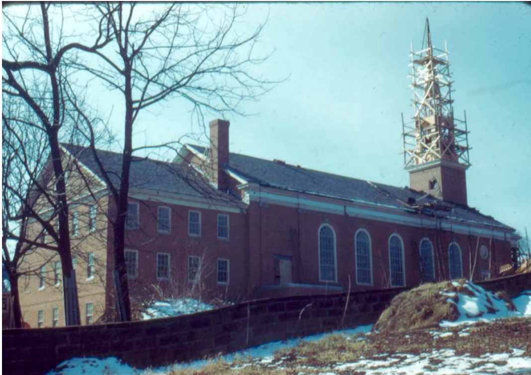
Park Street Church under construction 1956
