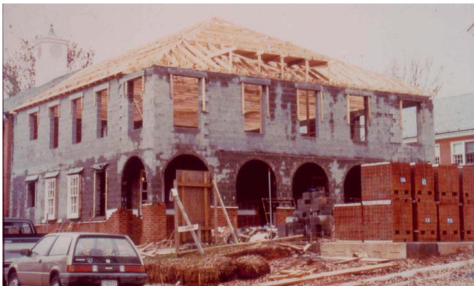
Educational Wing Construction, 1987
